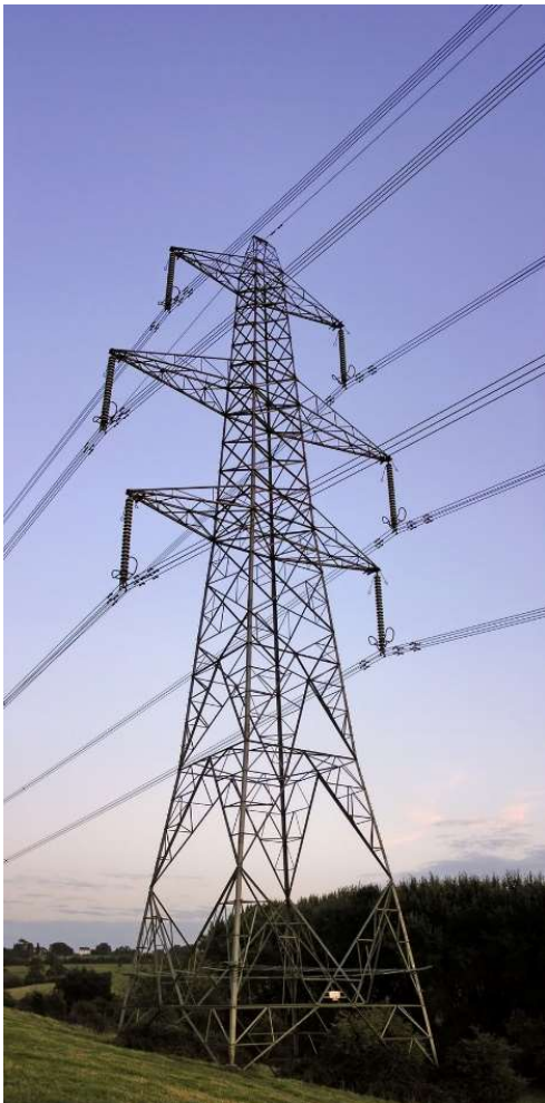
Image 4.1 - Typical suspension steel steel lattice pylon
