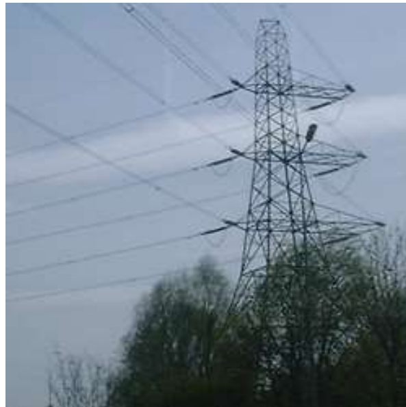
Image 4.2 - Typical tension/angle lattice pylon
